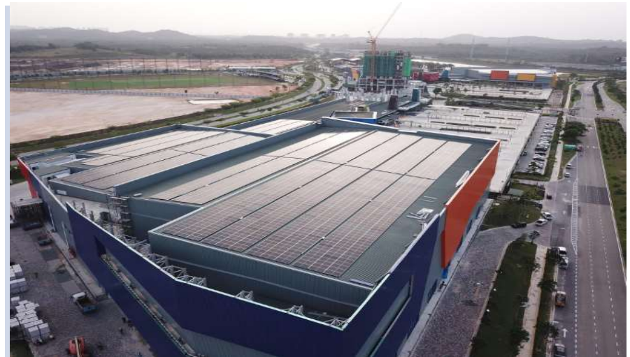
Roof Top Solar – Sunway Iskandar
